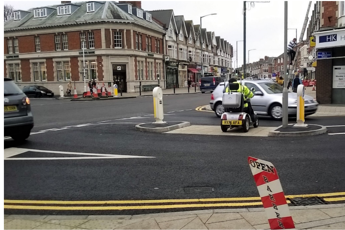
Bournemouth. 'New' side-road configuration. Designed 2016.
