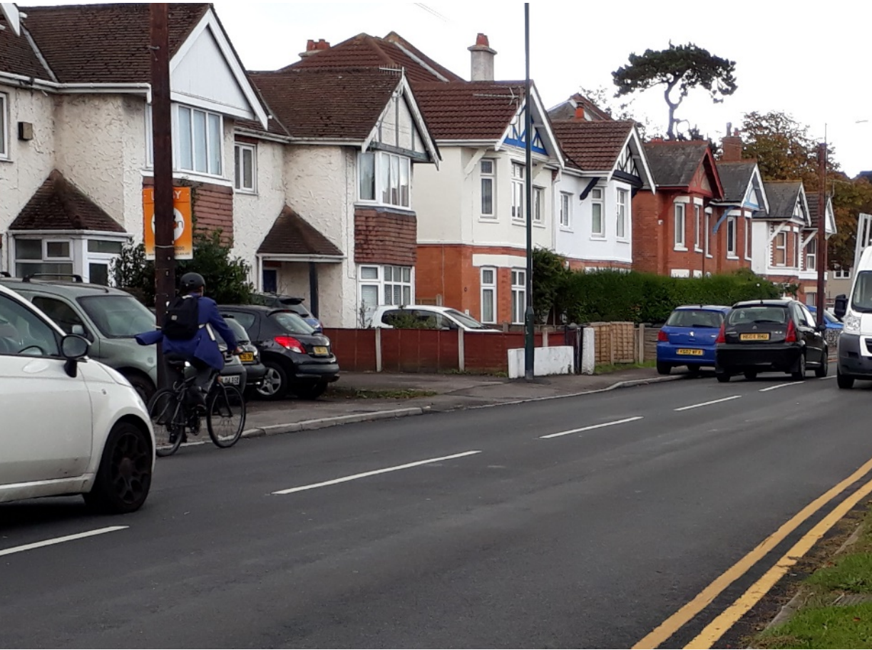
Bournemouth, UK. Road re-surfaced in 2017.
