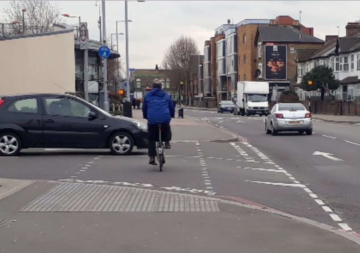
Tottenham Hale, London. Constructed c. 1990?
