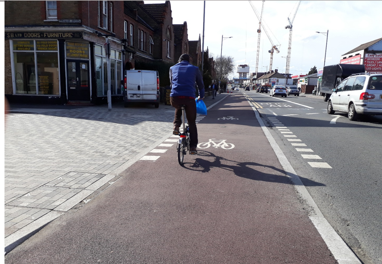
Lea Bridge Road, London. Constructed 2018
